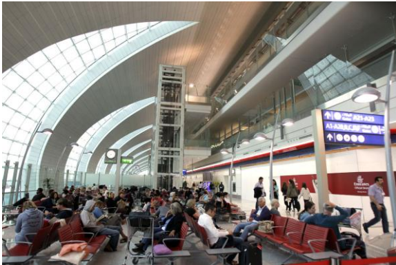
Fig. 3: Departure lounge in Concourse A at Dubai International Airport. The KNX-based lighting control system is linked to the flight schedule.
