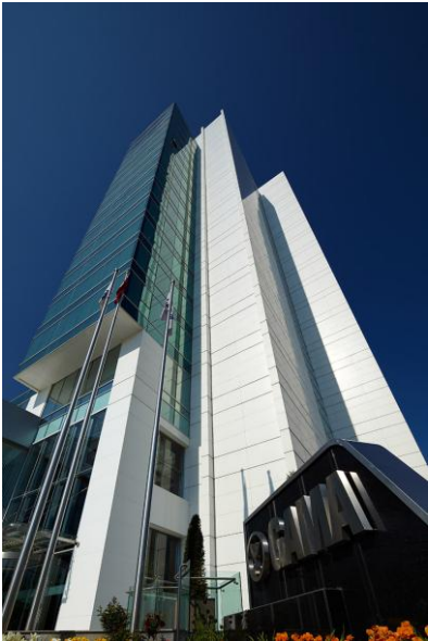
Fig. 2: At the GAMA headquarters in Ankara, KNX makes sure that electricity, gas and water are used as efficiently as possible.
